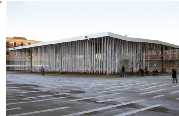
Ropes hanging from a structure formerly used to shelter a vehicle refueling station, former Carlsberg Brewery, Copenhagen, 2011. Photo: Brett Bloom
