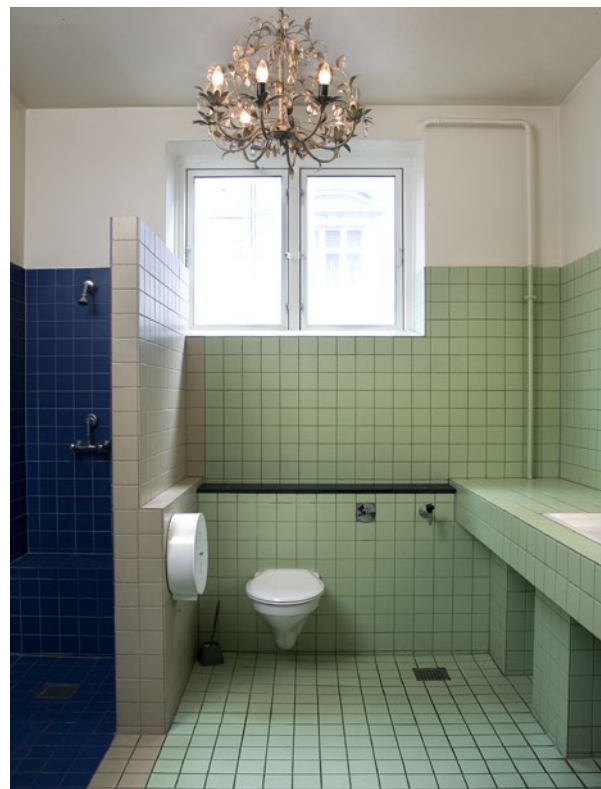
The new toilet got closed due to too much succes. It was used as an injection room.
