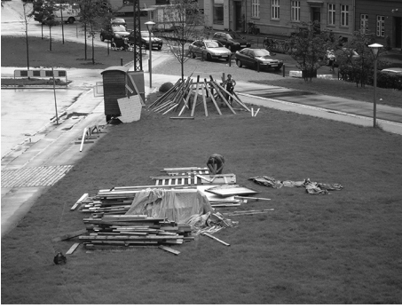
Figure 1.1. Beginning the process of construction.
